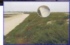
Example of natural return of vegetable cover after the implementation of a STABIPLAGE® established longitudinally at the bottom of the dune.
