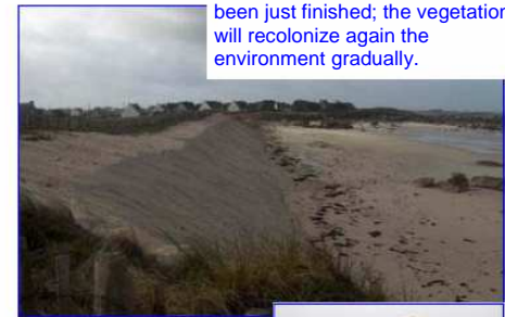
Example of natural return of vegetable cover after the implementation of a STABIPLAGE® established longitudinally at the bottom of the dune.
